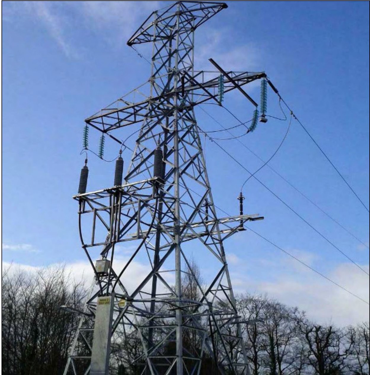
Figure 2.4 Photograph of a 110kV earthwire line/cable interface mast (used whenever a circuit converts from an overhead line to an underground cable).
