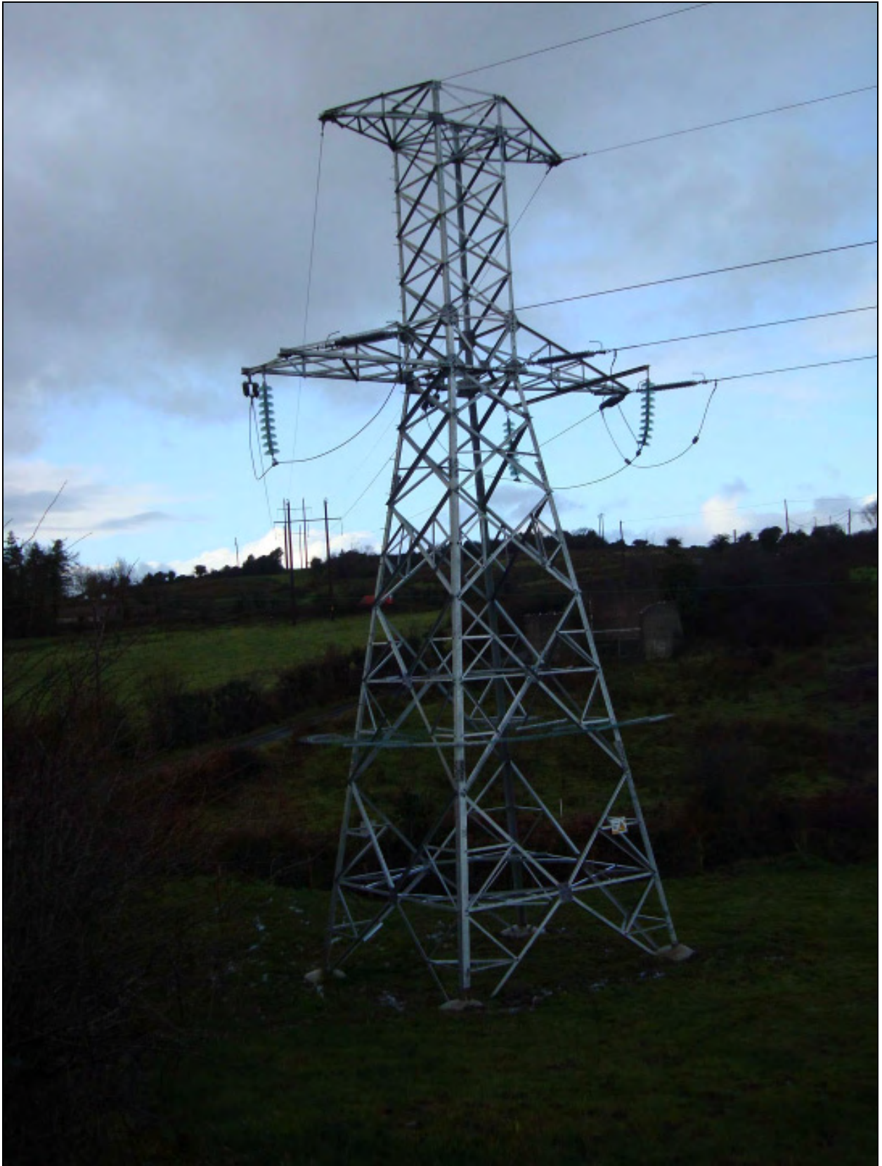
Figure 2.7 Photograph of a 110kV earthwire angle mast (used wherever a 110 kV overhead line changes direction).
