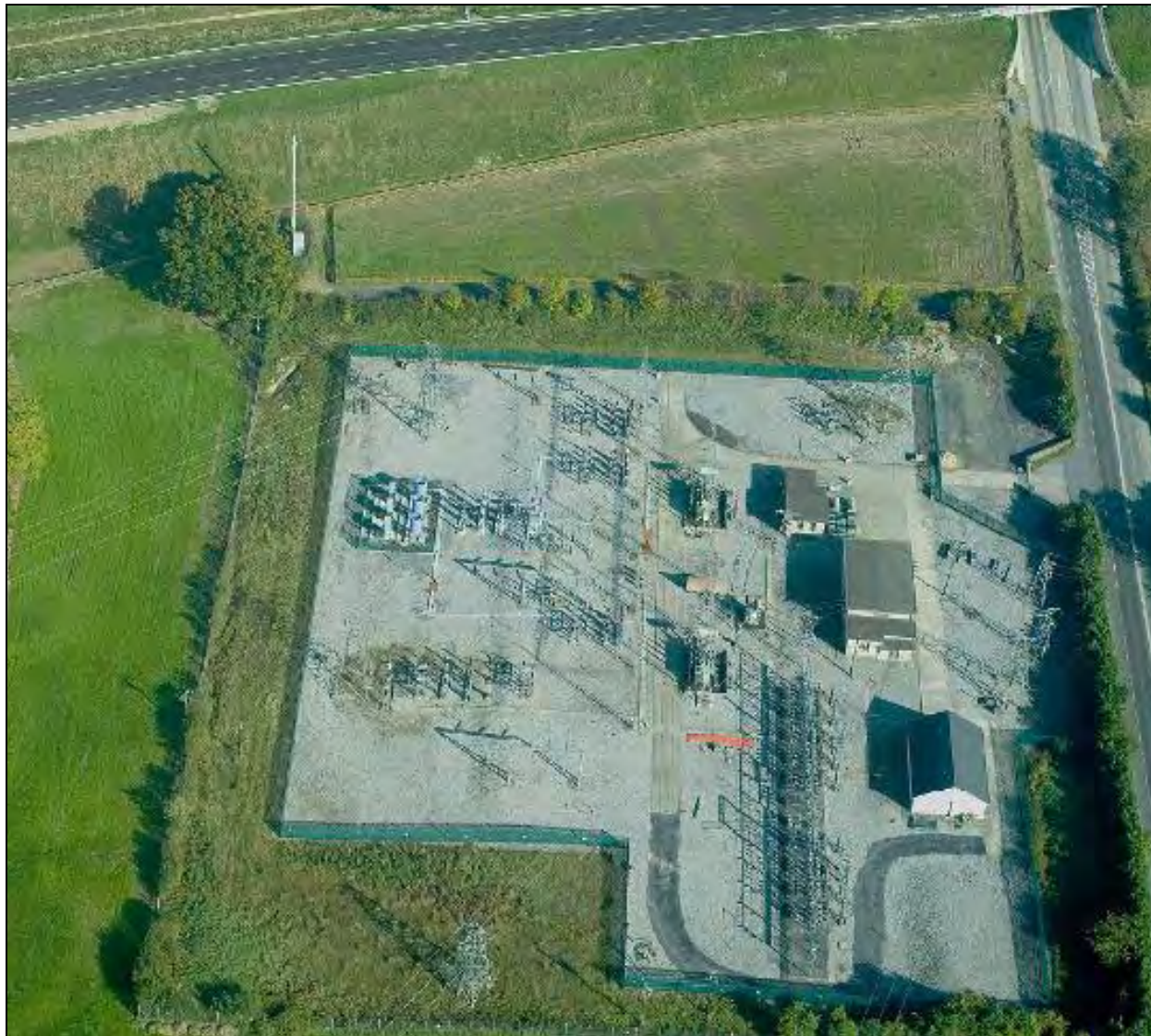
Figure 2.11 Photograph of Kilkenny sub-station; the location of proposed development unit 7 is at the furthest bottom left corner of the compound.
