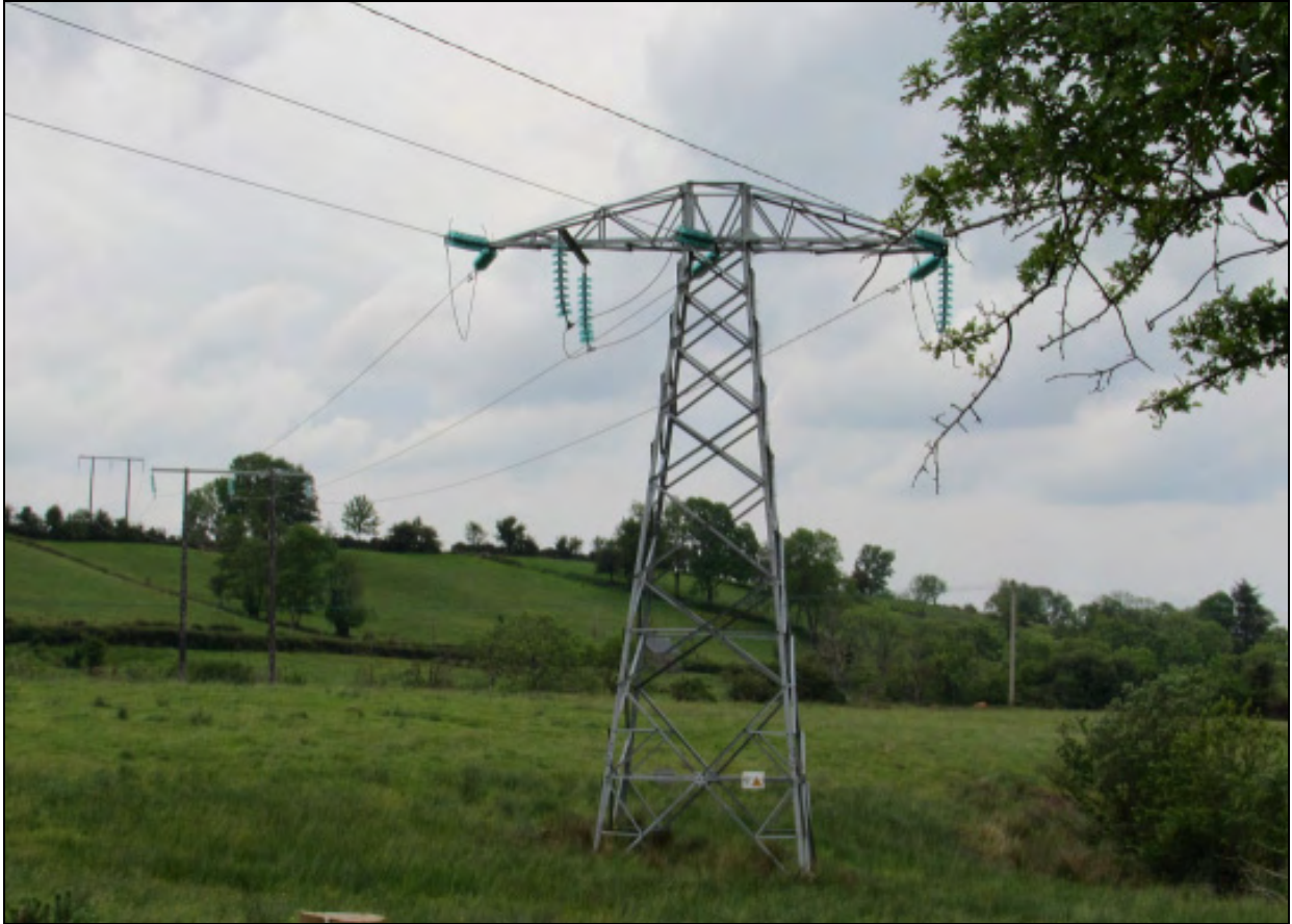
Figure 2.9 Photograph of a 110kV non-earthwire angle mast
