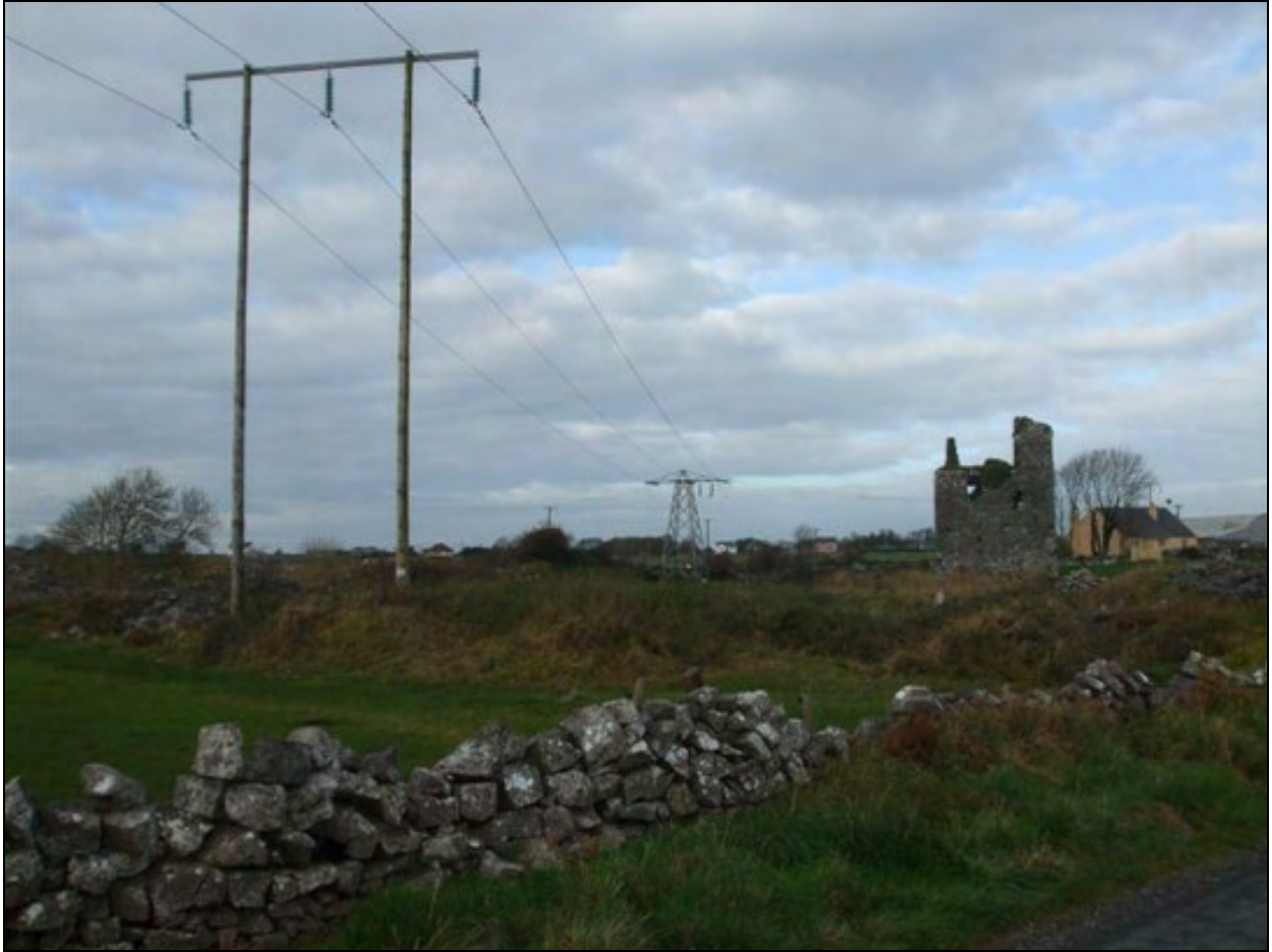
Figure 2.10 Photograph of a 110kV non-earthwire poleset
