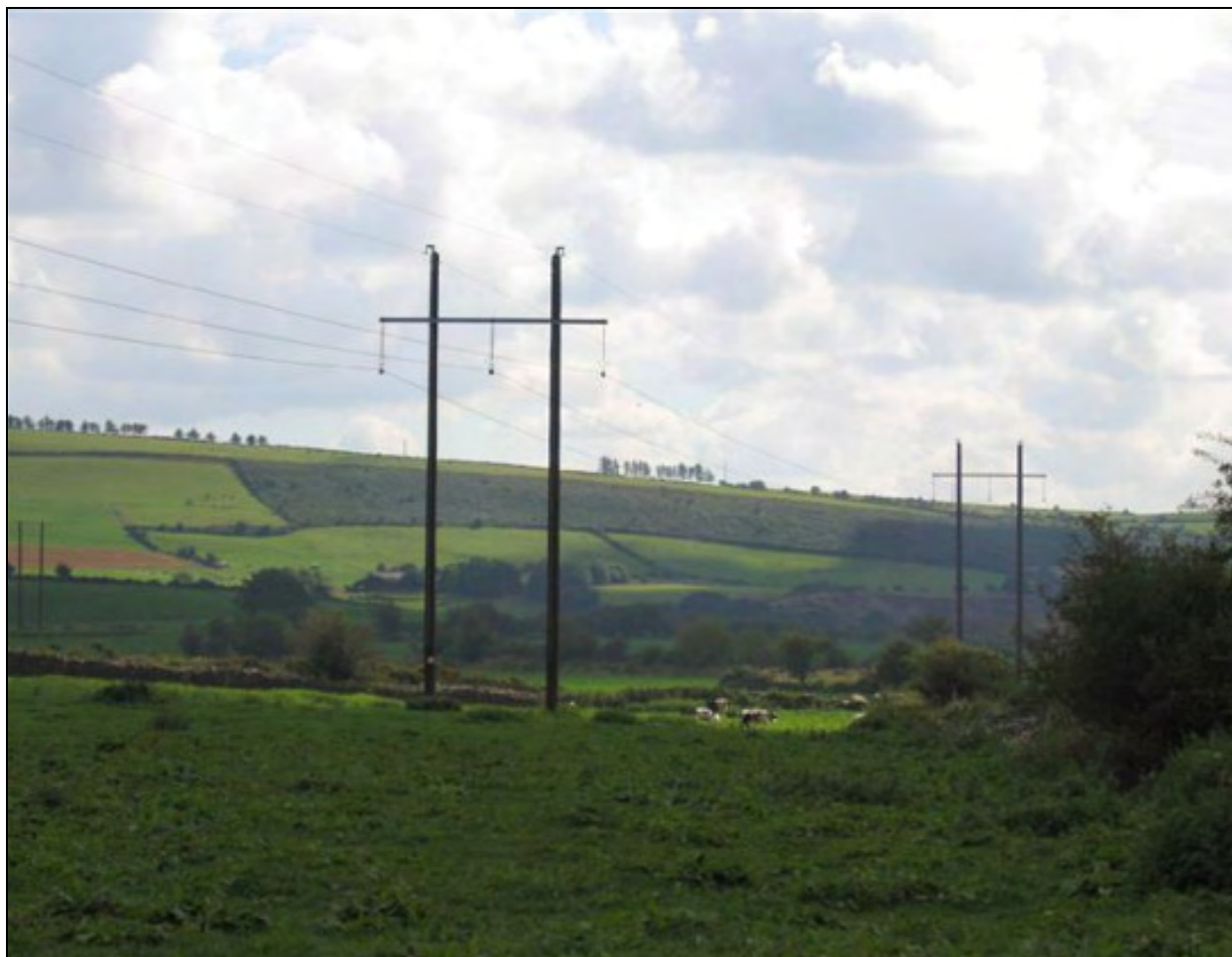
Figure 2.8 Photograph of a 110kV earthwire poleset
